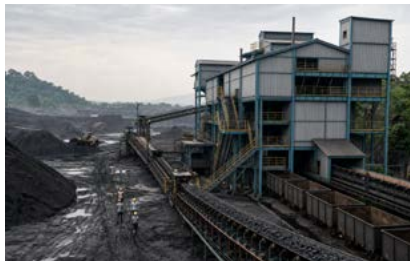
Coal washery, Raigarh
